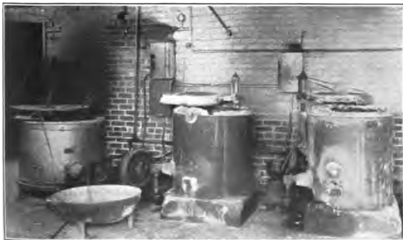
B. OIL FURNACES FOR REDUCTION OF SULPHATES AND REFINING OF SODIUM URANATE.
